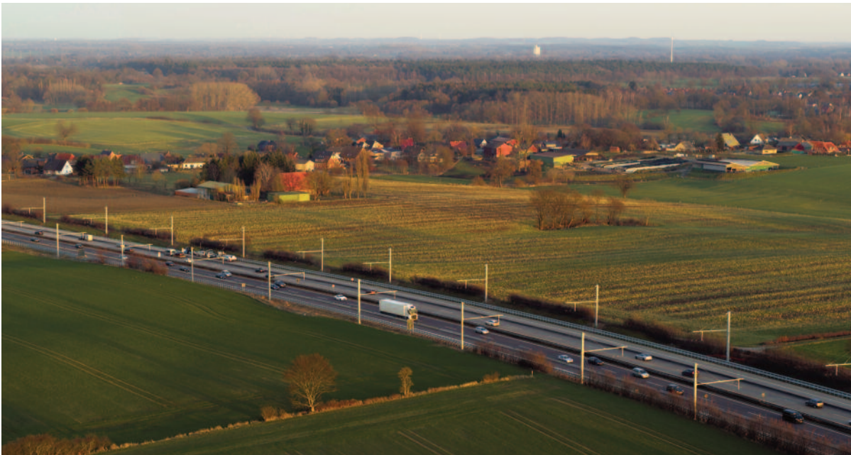
The third eHighway in Germany is also the longest so far. Overhead wires were installed on a five-kilometer section of the A5 federal Autobahn between the Zeppelinheim/Cargo City Süd interchange and at the Frankfurt Airport and the Darmstadt/Weiterstadt interchange. Following a test period, the decision will be made on whether to extend the system.
