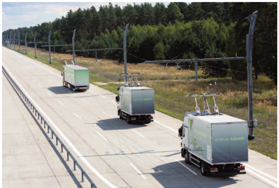
Multiple trucks can use the eHighway at the same time. In fact, the system makes use of regenerative braking where a vehicle braking or going downhill can add power back into the system for other vehicles to use. A fourth test eHighway is now under construction on the Autobahn A1 in the north of Germany.
