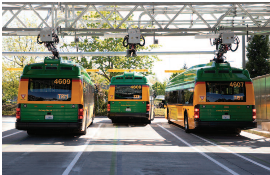
King County Metro Transit in Seattle recently selected Walsh-Stantec to assist with their transition to a zero-emission bus fleet. The project includes parking and charging stations for 120 ZEB buses at King County's Interim South Base in Tukwila. King County operates a fleet of 1,400 buses and serves a population of more than 2.1 million people.
