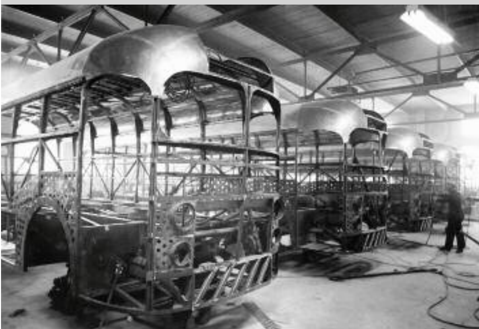
In 1940, the company was renamed Motor Coach Industries and moved to a larger facility. The new location at Erin and St. Matthews streets had 20,000 square feet that could better handle increasing production. This photo shows a series of coaches being built on what was then the assembly line.
