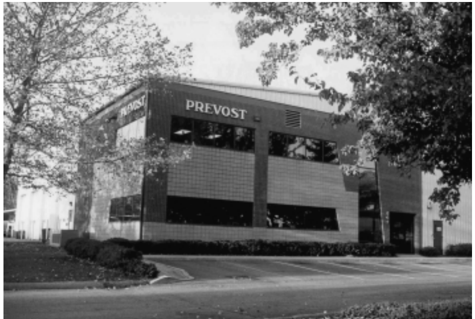
The facility in Lyndhurst, New Jersey is Prevest's oldest service center. In addition to offering parts and service, the building also houses Prevest's corporate office in the United States. It is located just north of Newark and just across the river from New York City.
