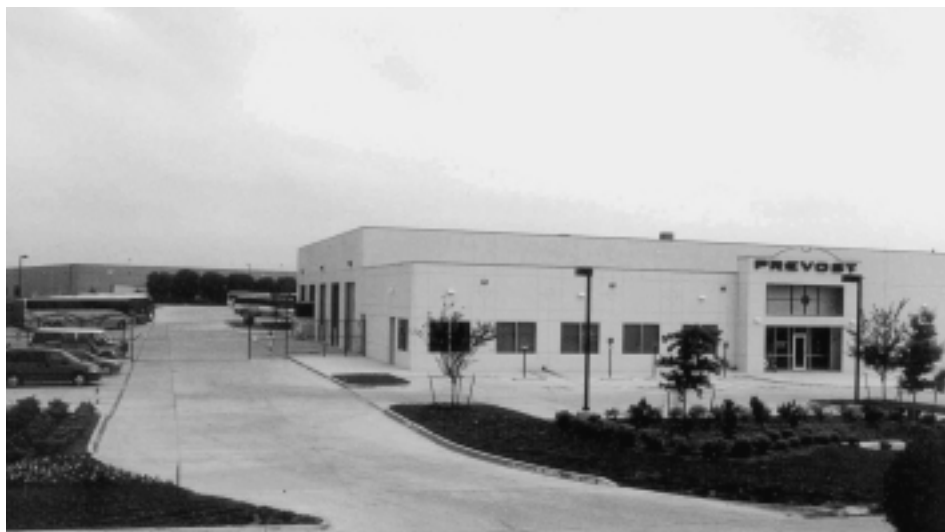
The Fort Worth facility is Prevost's newest service center. It is located south of Dallas-Fort Worth International Airport in a modern industrial park. There is plenty of room here with more than 100 bus parking slots and 14 spots with plug-ins for converted coaches.
