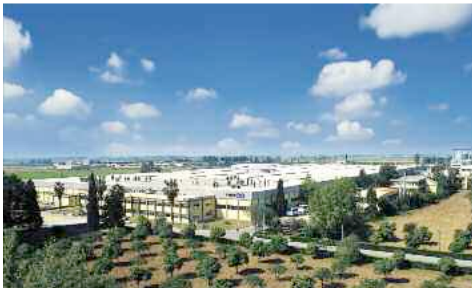
Temsa's major bus factory is located on the west side of Adana, Turkey, about 600 miles southeast of Istanbul and a few miles north of the Mediterranean Sea. It is located on 110 acres and has approximately 1,500 Temsa employees with another 500 who work for suppliers. TEMSA.
