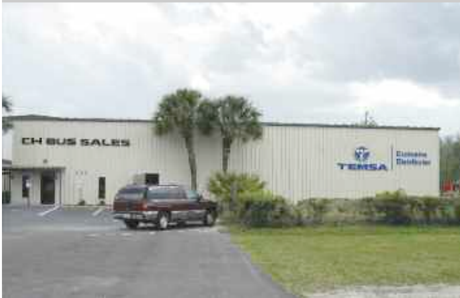
The new facility of CH Bus Sales is located at 410 W. Taft-Vineland Road, just west of the Orlando airport. In addition to five bus bays, the facility has a 5,000-square foot parts warehouse. New coaches are prepared here for customer delivery. CH BUS SALES.
