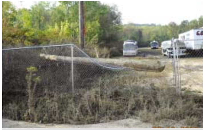
This utility pole fell across the Annex fence during the flooding. The Annex still did not have power two weeks after the flooding. There was similar damage around the immediate area. JOT BENNETT.
