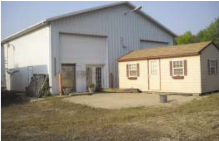
Taken on September 13, this photo shows that there is no serious damage to the Annex building or office. With some power washing inside and out, it can return to regular use. JOT BENNETT.
