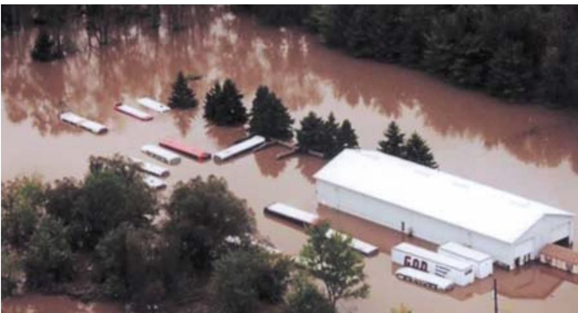
This photo shows the Annex building and surrounding parking area at the high point of the flooding. The floodwaters covered everything but the roofs on some of the buses. Even those buses inside the building were sitting in a few feet of water. GEORGE HERWIG.
