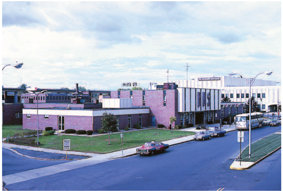
The new Springfield Bus Terminal at 1776 Main Street opened in 1969. In addition to being a terminal it also served as a corporate office and maintenance facility. Regular bus operations moved out to Union Station in 2017 and the offices followed a year later.
