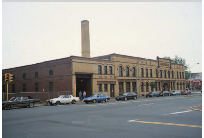
The old 1897 Trolley Barn in Springfield was acquired in 1958 and served as the Peter Pan garage and office for years. It was later turned over to Coach Builders, Inc. and used for doing bus repair work.
