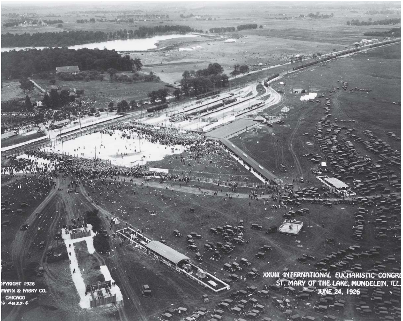
This overhead photo looks northeast and shows the temporary terminal at the seminary in the center of the photo. The double track main line of the North Shore Line is just north of the temporary terminal. The temporary bridge across the North Shore Line main line is just off of the photo to the left while some of the auto parking area can be seen at the lower right. Those with sharp eyes might see a couple of cars parked on the main line as well as numerous people along the road to the north of the tracks, presumably walking from the Milwaukee Road at Libertyville. UNIVERSITY OF ST. MARY OF THE LAKE ARCHIVES.
