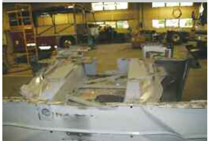
The biggest problem with collision repair is hidden damage. This "bogie" frame at the front wheels was replaced rather than pushed back into shape because of extensive damage.
