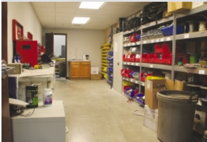
The new electrical room not only provides a stock of various electrical components, connectors and wires but also offers a clean area for working on electrical components.
