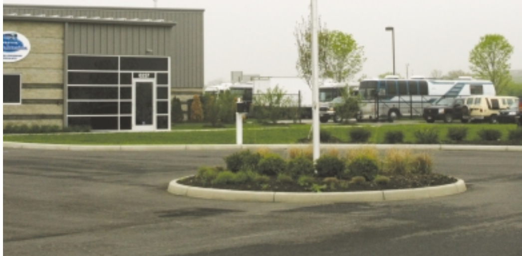
The completion of the new conversion facility for Creative Mobile Interiors in Grove City, Ohio coincides with the company's 10th anniversary. All operations, including conversion work, upgrades, repairs, rebuilding and vehicle service work are now under one roof. This photo looks almost south with Interstate 71 to the right behind the parked coaches and the main entrance to the new building in the center.
