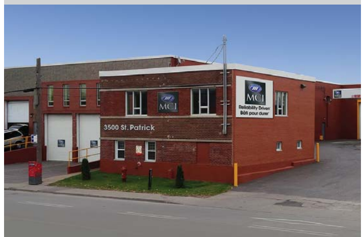
MCI recently moved its Montreal service center to a new location that is larger and more modern. It is open 24/7 and offers a wide range of services.
